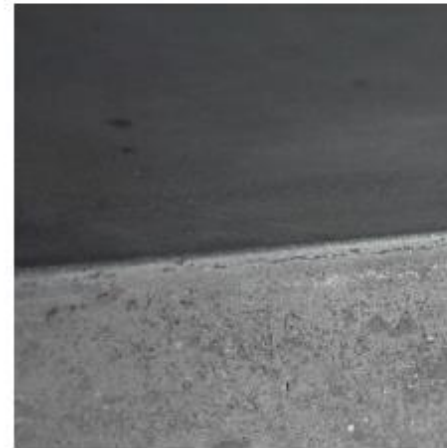
Seams and mold impressions create color variations.
